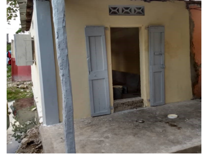
Outside of Mrs. Seide's home in Les Cayes, on November 22, 2022
