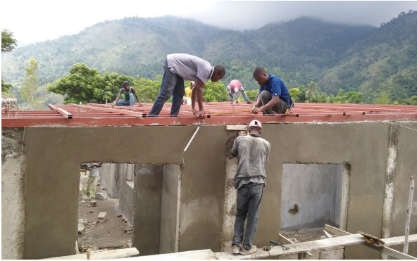
Photo (Above): Construction of M.V. school - Aug. 16, 2016.
